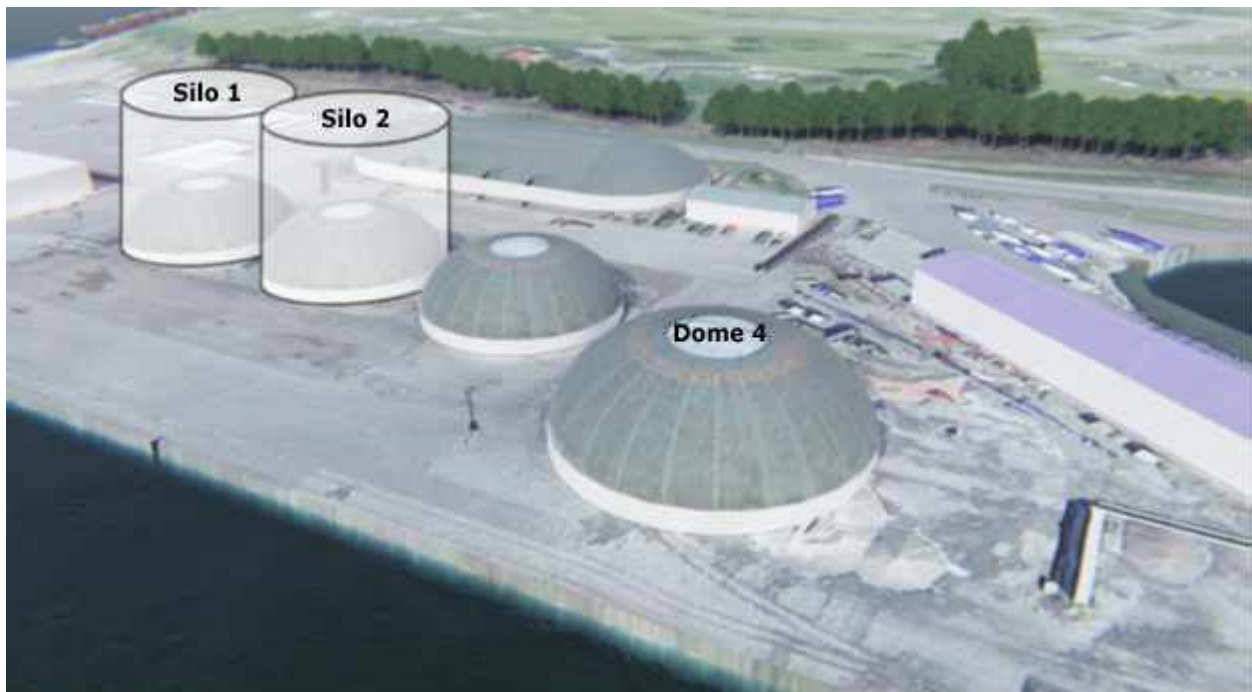
Silos 1 and 2 replacing existing Domes 1 and 2 and new Dome 4.
